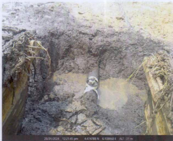
Incident point with 3" Valve Installed
