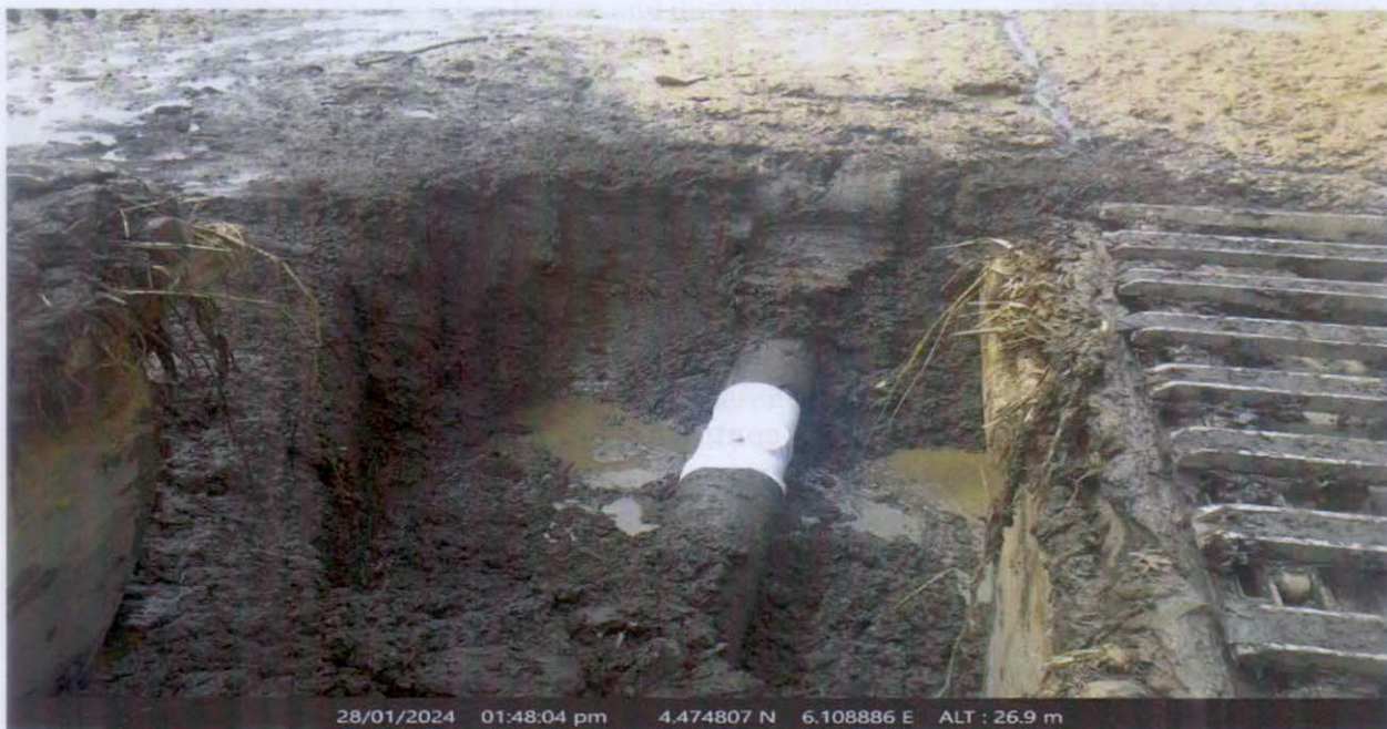
Repaired incident point
